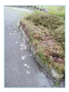
Concrete curbs appear to be deteriorating at a rate typical of their age. This repair contingency has been included due to the likelihood of additional damage from roots and vehicles.
