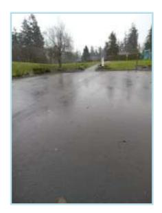
Appears to be deteriorating at a rate typical of its age. As routine maintenance, keep surface clean, ensure that drains are clean and free flowing, repair cracks and clean oils stains promptly. Best to plan for eventual intervals of resurfacing (overlay).
