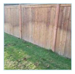
Wood fencing (at Snohomish Cascade Drive) appears to be deteriorating at a rate typical of its age. As routine maintenance, inspect regularly for any damage, repair as needed. Avoid contact with ground and surrounding vegetation. Regular cycles of stain/paint will help to maintain appearance and maximize life. Plan to replace at roughly the time frame indicated.
