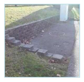
Masonry retaining walls on site appear to be in generally fair and stable condition; no significant instability noted. We assume that retaining walls were designed and installed properly with adequate base and surrounding drainage. Monitor closely and if areas of instability emerge, consult with civil or geotechnical engineer for repair scope.
