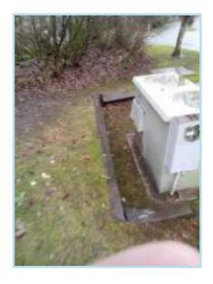
Wood retaining walls on site appear to be deteriorating at a rate typical of their age. We assume that these were designed and installed properly with adequate base and surrounding drainage. Monitor closely and if areas of deterioration emerge, consult with civil or geotechnical engineer for repair scope.
