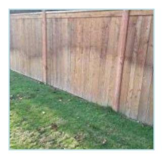
Regular sealer applications (stain/paint, etc.) on the timeline indicated are strongly recommended for appearance and protection of wood fencing. Remove any contact with ground and surrounding landscape and sprinkler patterns, repair as needed and clean prior to sealer application. Life of finish will vary depending upon surface preparation, material quality, application method and weather conditions.
