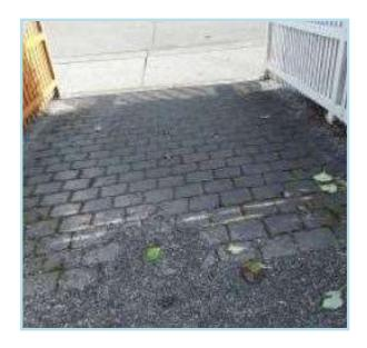
We recommend budgeting for replacement at the timeframe indicated as these sand set paver systems will typically become uneven with time due to settling, root intrusion, drainage issues and use.
