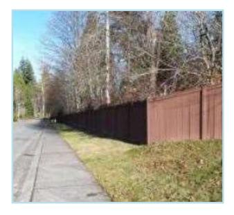
Wood fencing (at NW Pond) appears to be deteriorating at a rate typical of its age. As routine maintenance, inspect regularly for any damage, repair as needed. Avoid contact with ground and surrounding vegetation. Regular cycles of stain/paint will help to maintain appearance and maximize life. Plan to replace at roughly the time frame indicated.
